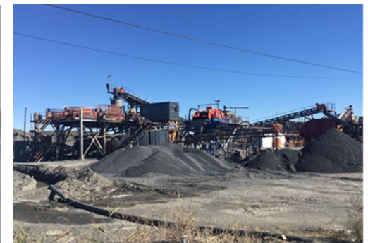
Bulk Sampling Plant
